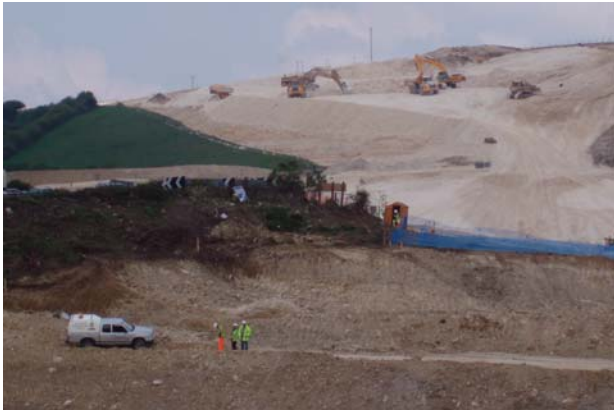
Purbeck Beds exposed in an excavation for the northern foundation of the arch bridge at Bincombe.
