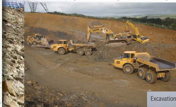
Excavation in progress in the cutting at Southdown Ridge
